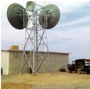
Check buildings and assets
